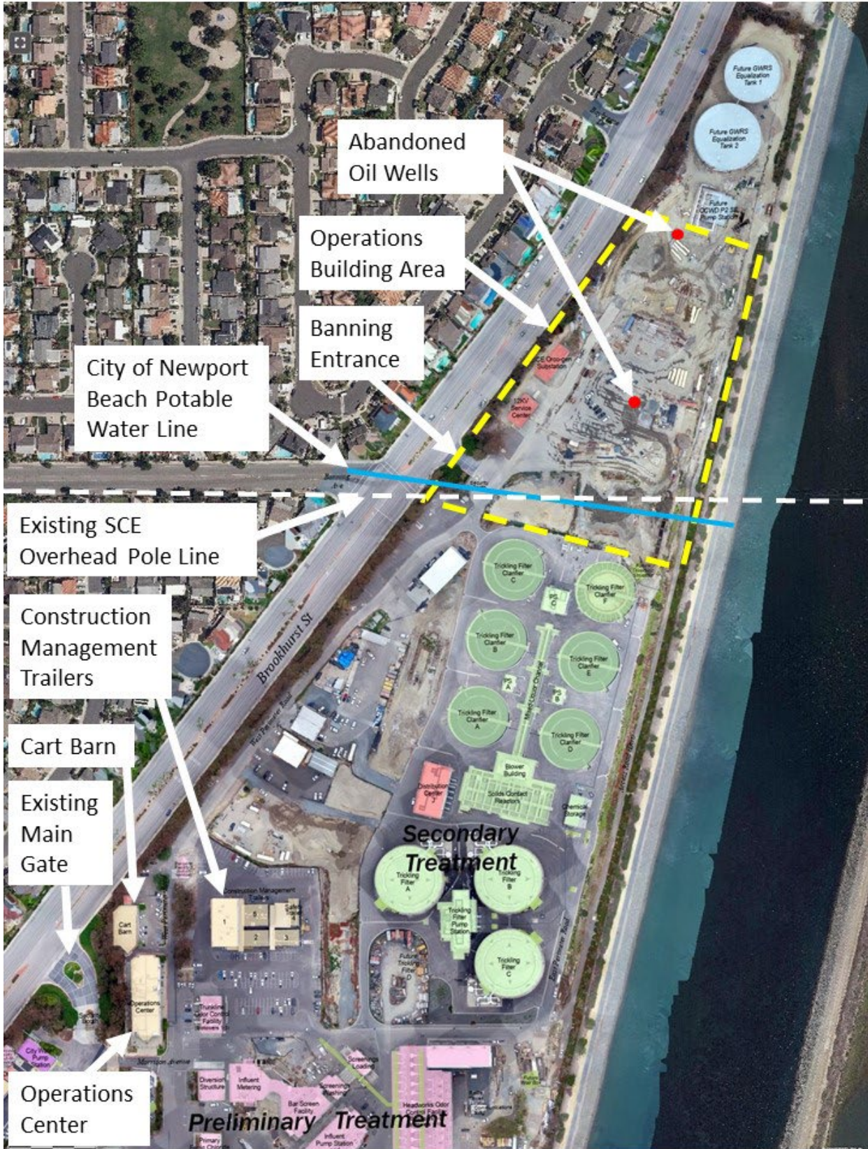
Figure 1 – Plant No. 2 Project Site
