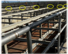
Replace handrails at secondary clarifiers
