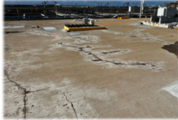
Rehabilitate aeration basin deck
