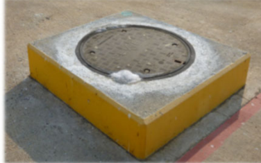
Seal leaking manholes
