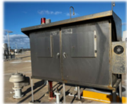
Add air conditioning to control panels
