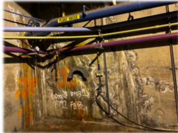
Rehabilitate concrete in tunnels
