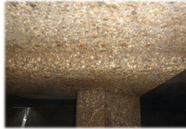
Rehabilitate interior of aeration basins
