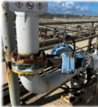
Replace oxygen piping
