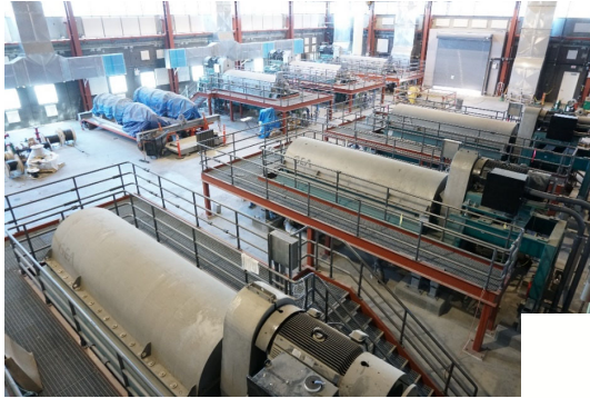
Centrifuge System at Plant No. 1
