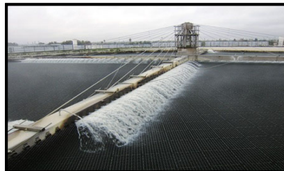
Trickling Filter at Plant No. 1
