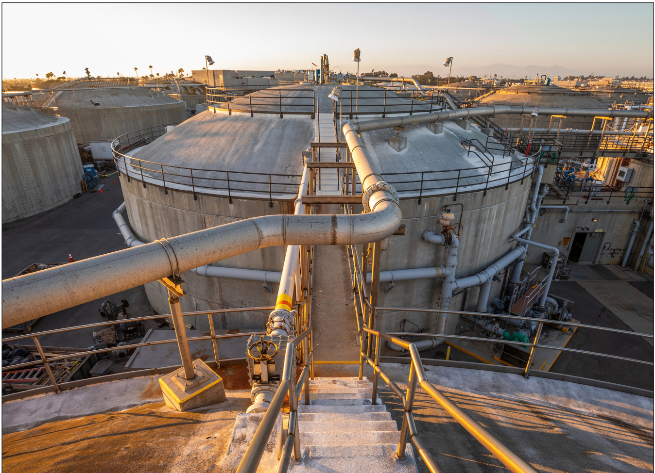
Digesters at Plant No. 2 in Huntington Beach.
