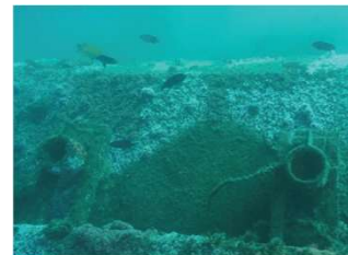
End Structure Flap Gate Hinges
