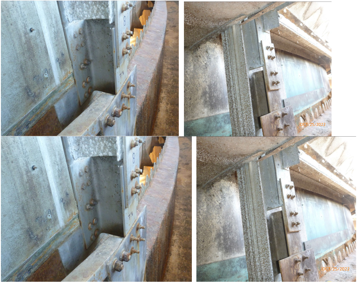
Figure 8: Dome post typical configuration in Clarifier G
