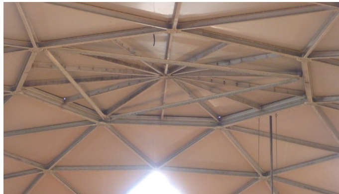
Figure 15: Aluminum stiffeners below the removable dome hatch
