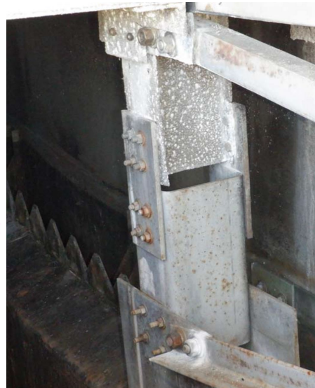
Figure 3: Retrofitted support post with new stainless-steel stub and plates in 1995
