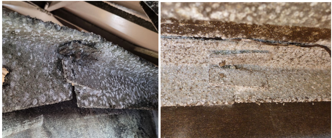
Figure 14: Connector between two aluminum angles
