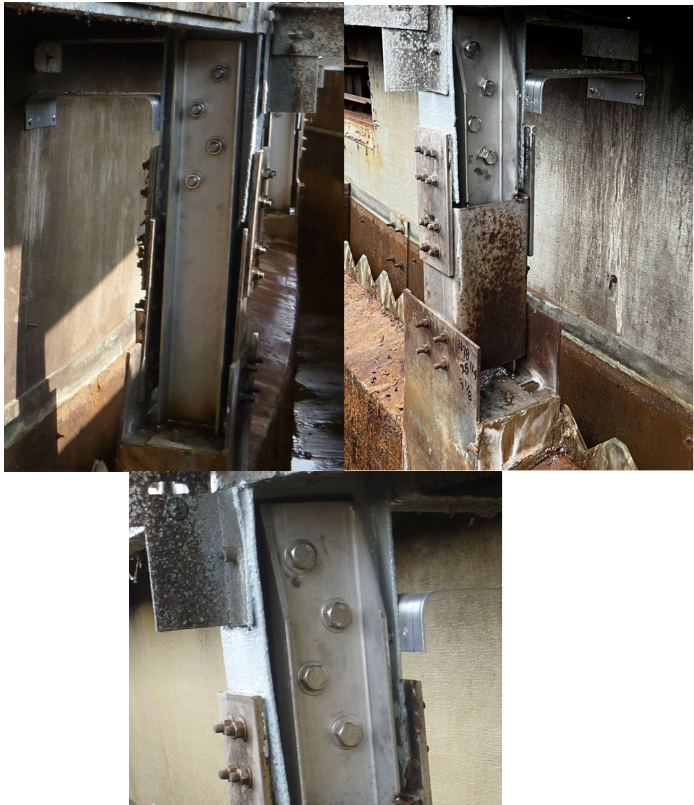
Figure 7: Reinforced dome post (different basin) (typical)
