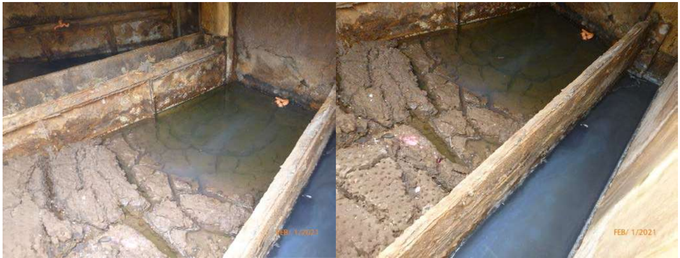
Picture 10: One of weir slabs for PSB-M, and channel below filled with primary influent. Sludge on top of slabs will be removed by OC San.
