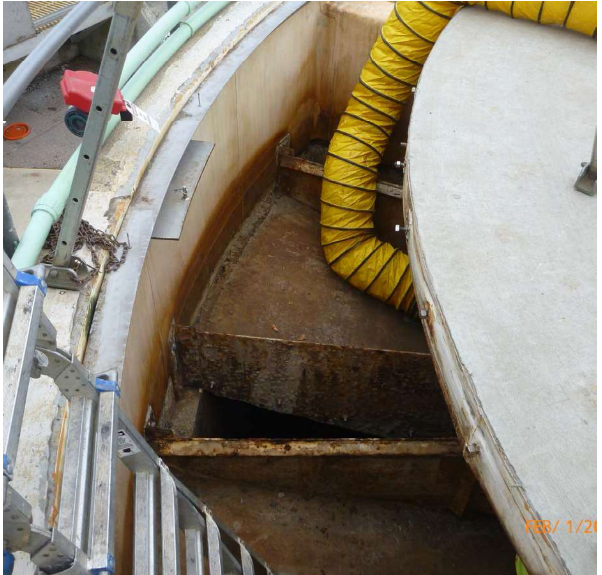
Picture 11: FRP covers removed to access weir plates
