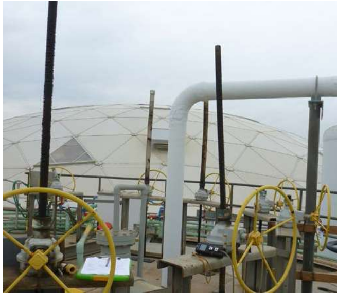
Picture 3: Bent stems and bevel gear operators
