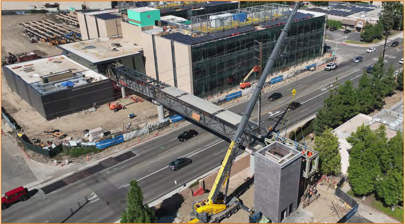
Construction of new 109,000 square foot, 3-story Headquarters building and pedestrian bridge.
