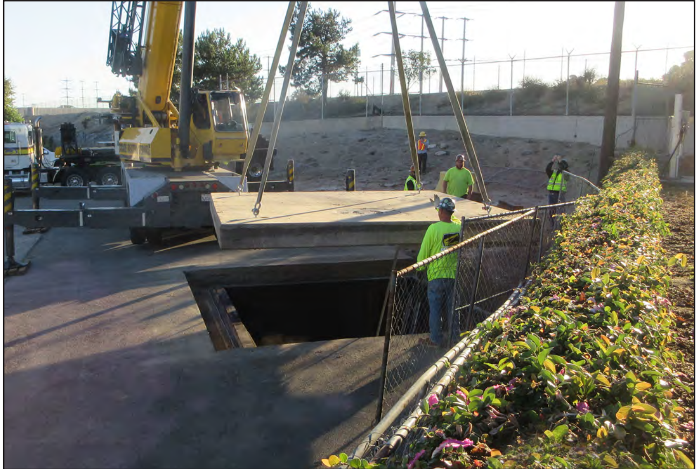
Removing manhole cover on the Santa Ana Trunk Rehabilitation at Plant No. 1 Project.
