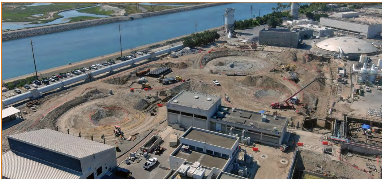
A-Side Primary Clarifiers Replacement at Plant 2 in Huntington Beach.
