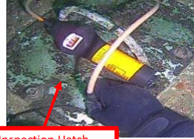
Inspection Hatch Pre/Post Cleaning and Thickness Testing
