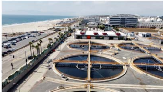
The Los Angeles Regional Water Quality Board is requiring Los Angeles to conduct additional offshore monitoring and to provide daily reports about ongoing discharges at the Hyperion Water Treatment Plant. Signs at Occidental State Beach across the street from the plant, advise people that contact with the water may cause illness. in Playa del Rey on Friday, July 30, 2021. (Photo by Dawn Magrino/Daily News, SCNG)
