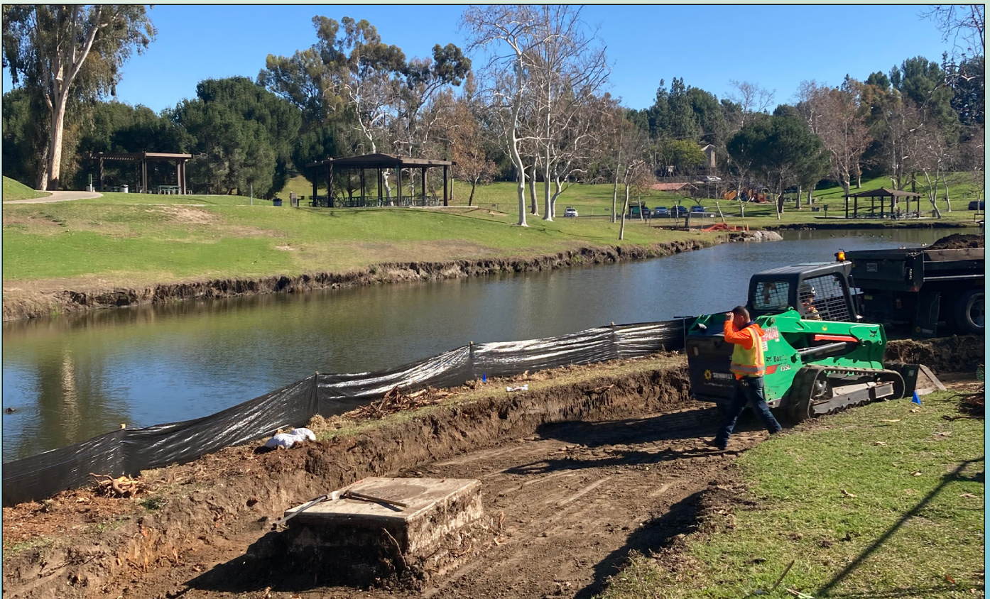
Crew preparing area for structural pavers.
