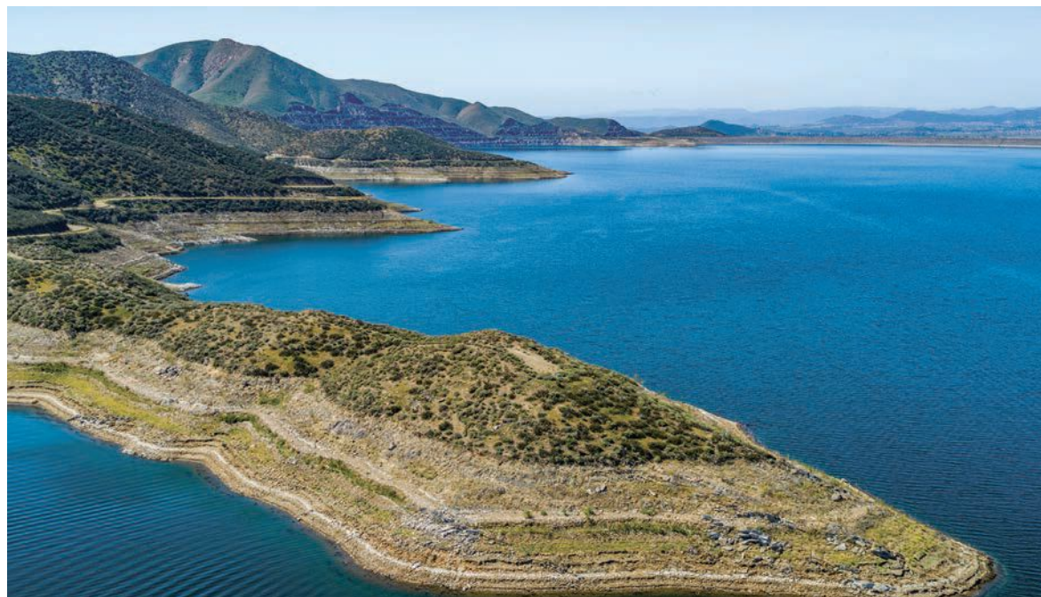
Above, Diamond Valley Lake in Hemet, built by Metropolitan, provides water storage close to home. Water agencies offer turf replacement rebates to encourage residents to plant drought-tolerant landscapes, as shown at right. Photos Courtesy of Metropolitan
