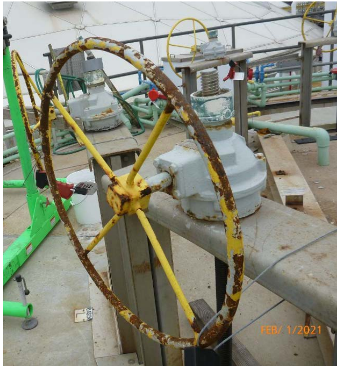
Picture 4: Corroded handwheel and bevel gear operator
