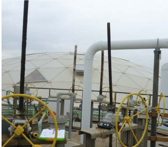
Picture 3: Bent stems and bevel gear operators
