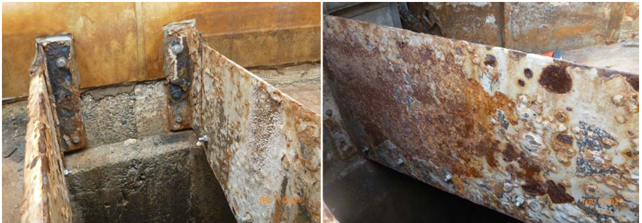
Picture 12: Corroded steel weir plates
