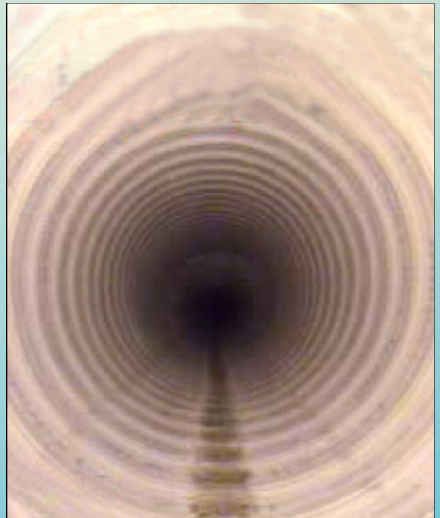
Cast iron pipe after installation of PVC liner.
