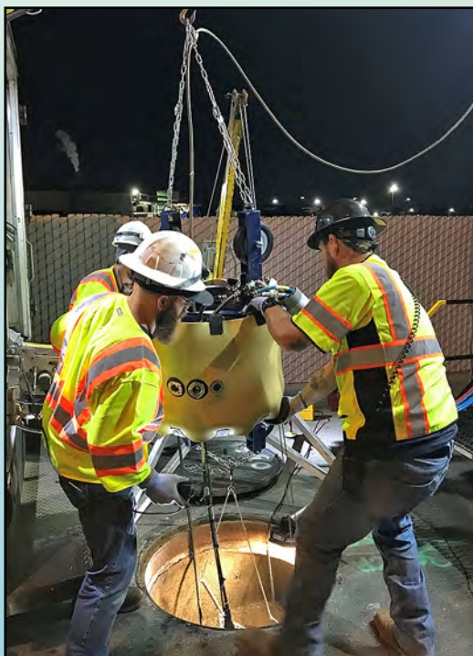
Contractor lowers the chemical grout injection packer into the manhole.
