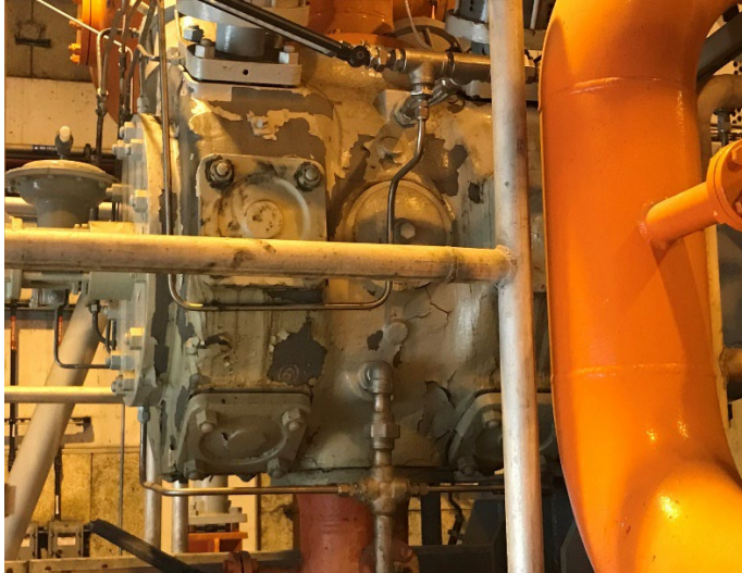
Figure 2: A Gas Compressor Cylinder showing signs of byproducts of corrosion and in need of replacement from a recent overhaul.
