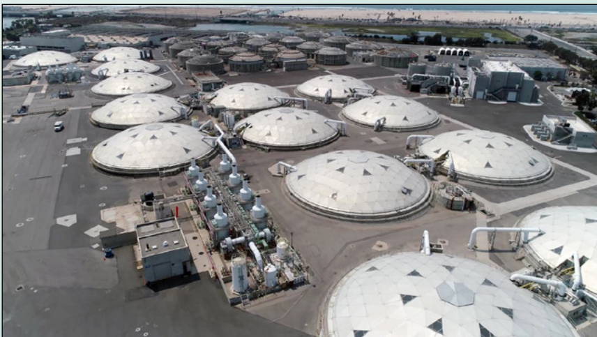
Aerial view of the existing Primary Clarifiers at Plant No. 2 in Huntington Beach.
