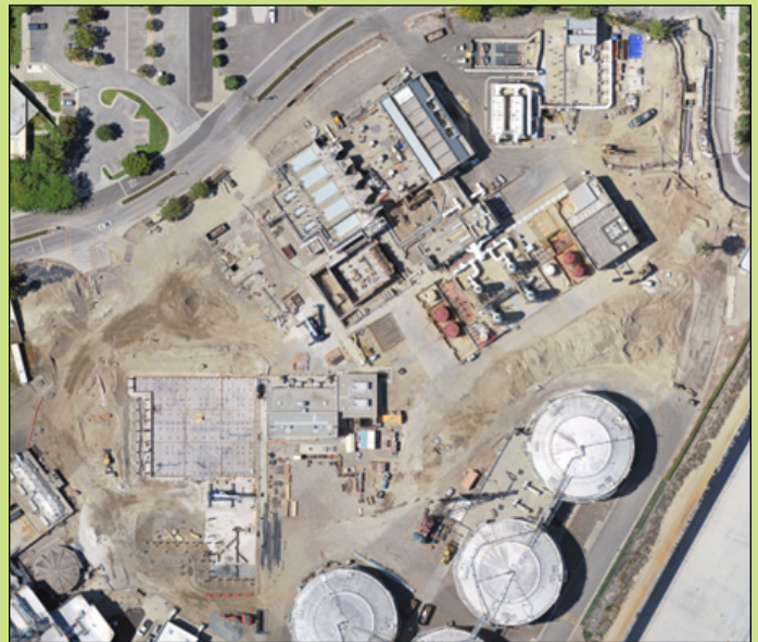
June 2022 – Headworks Project Progress
