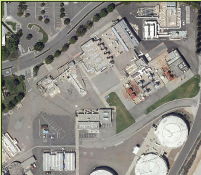
May 2021 – Headworks Project Progress
