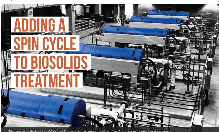
This project included the addition of five new dewatering centrifuges which replace the aging belt filter presses.
