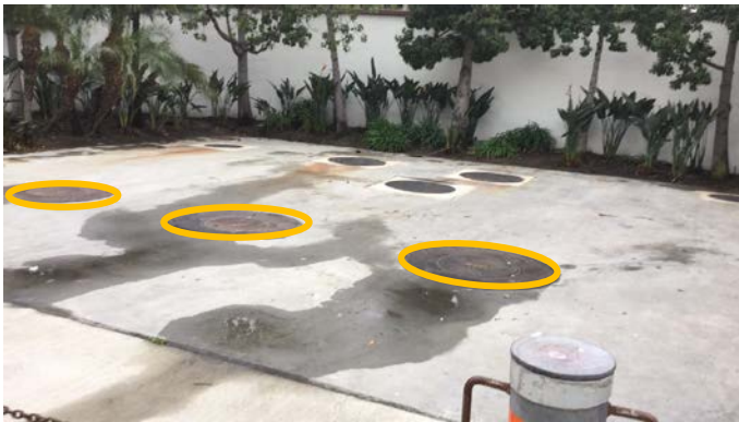
4 drywell hatches below flood level
