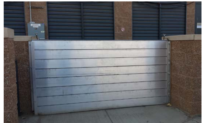
Stop logs over doors or sealed doors
