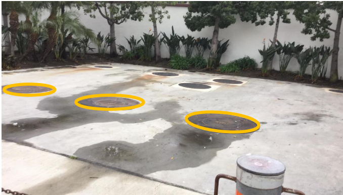
4 drywell hatches below flood level
