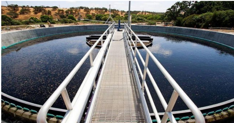
One of the new circular clarifiers at the Paso Robles sewage treatment plant, as pictured in May 2015.
