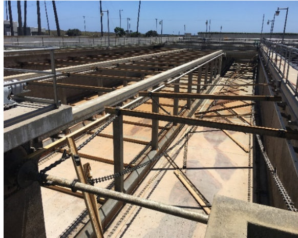
Broken Clarifier Mechanism
