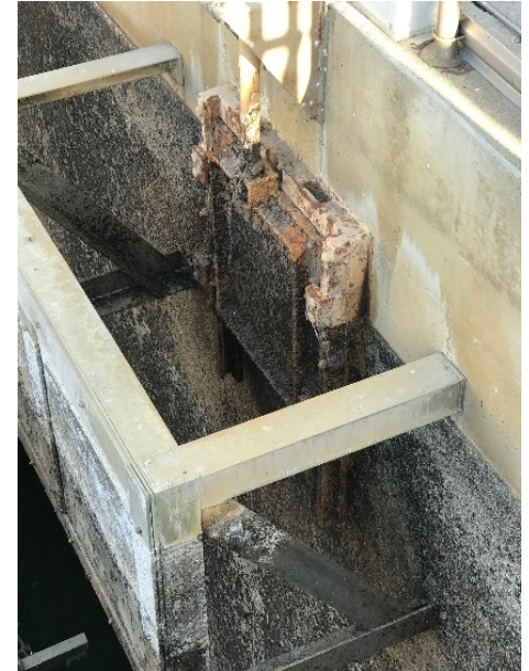
Corroded/Broken Inlet Gates
