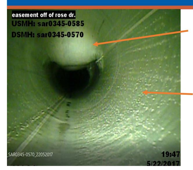
Sag where top of pipe collapsed during lining
