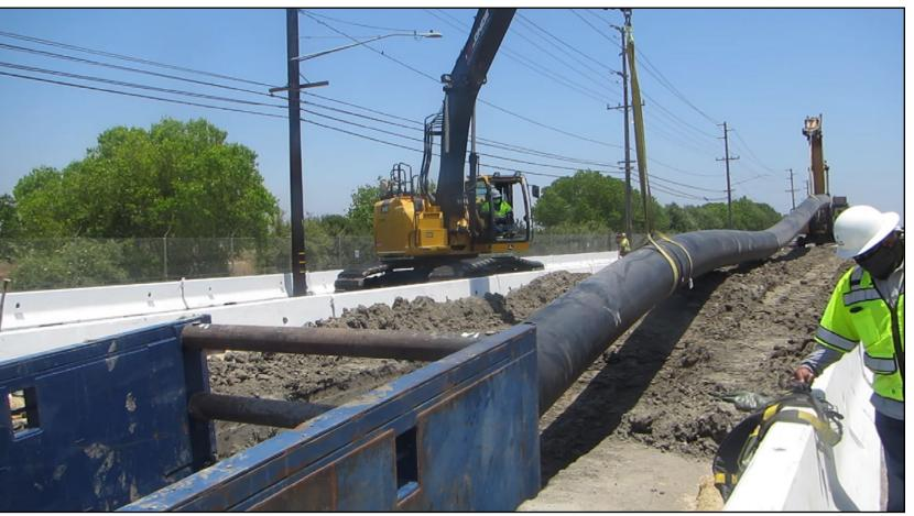
Two excavators are used to install a 200-ft section of a new 36-inch diameter force main within the 10-ft deep trench excavation on Westminster Boulevard in the City of
