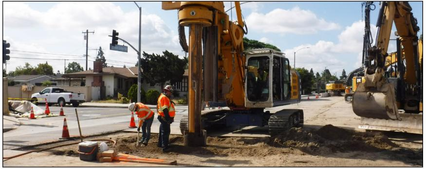
Construction crew is shown pre-drilling a shoring beam on State College Boulevard in the City of Anaheim.
