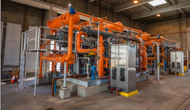
Digester gas compressor at OCSD Plant No. 1 will be replaced as part of the Digester Gas Facilities Replacement project.
