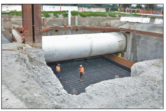
Excavation and shoring over the 120-inch diameter secondary effluent pipeline at OCSD Plant No. 2 in preparation for the plant water pump station junction structure.
