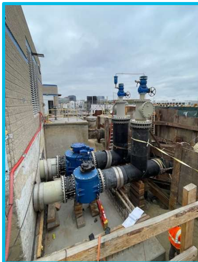
Valve Vault Replacement
