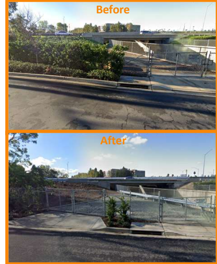
Manhole Access Improvements
