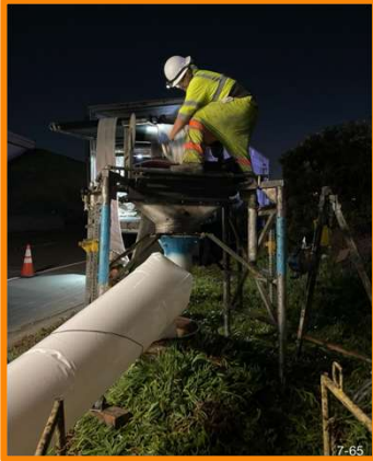
Gravity Rehabilitation Using Cured-in-Place-Pipe
